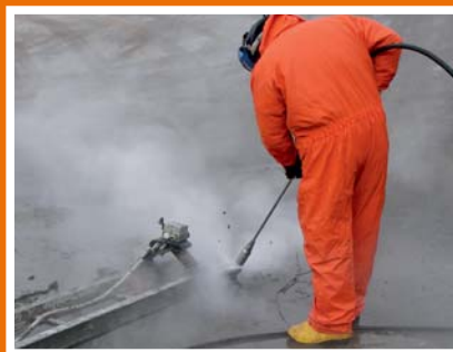
Removing concrete.
