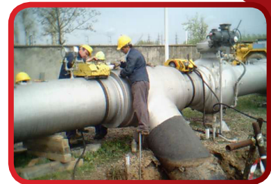
Trav-L-Cutter makes precision cuts facilitating section removal in the field
