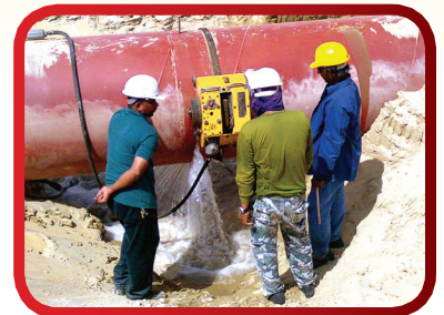
One Trav-L-Cutter can operate on multiple pipe diameters by adding additional chain sections
