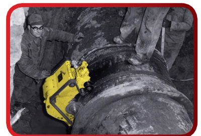
First introduced in 1949, Trav-L-Cutters are highly durable and in use all over the world
