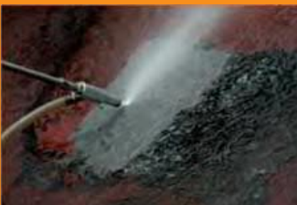
surface sand blasting
